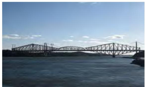
*Cantilever Quebec Bridge (rebuilt 1917)
